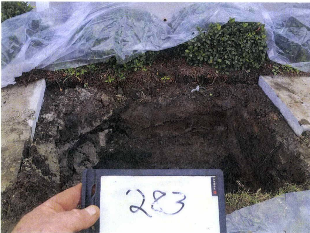
Picture 2: UST 283Birch excavation.
